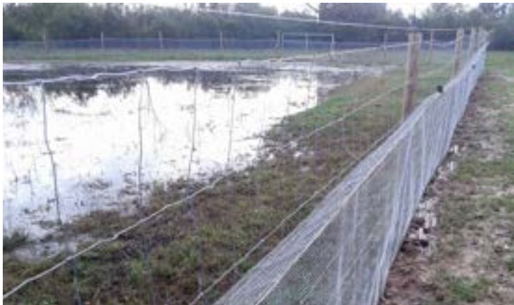
Figure 1.7. Knotted mesh fence to prevent access to wild boar and other ungulates, reinforced with an electro-welded mesh to block American mink from a high conservation value wetland area.
