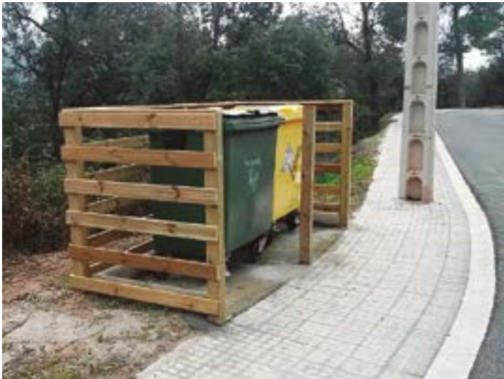
Figure 9.1. Containers with a partially screened perimeter to prevent wild boar from tipping them over.
