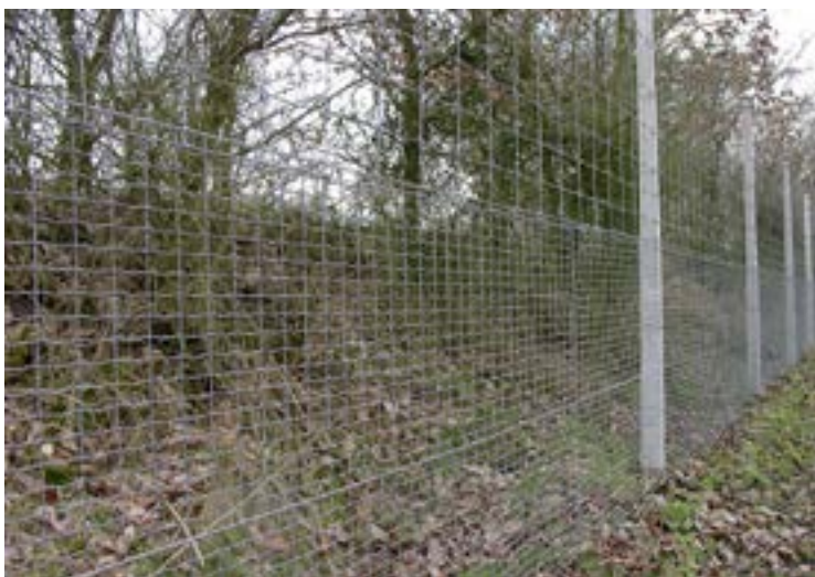
Figure 1.8. Fence combining electro-welded mesh for small fauna (lower part) with knotted mesh for ungulates (upper part).
