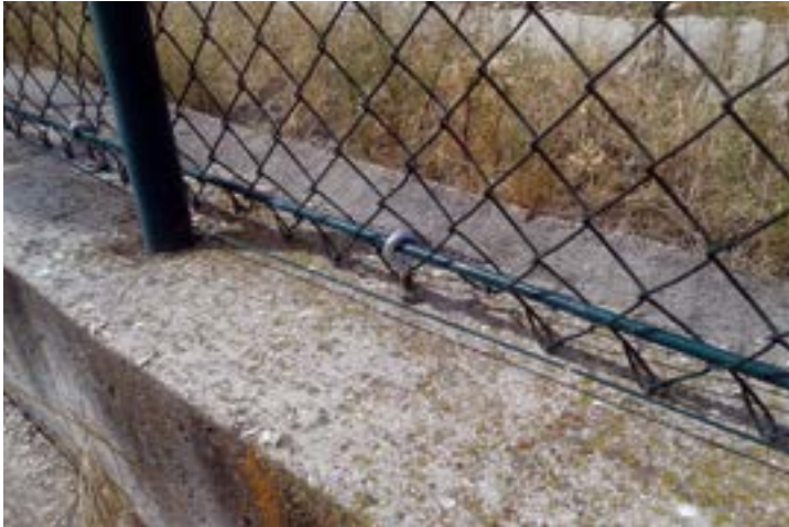
Figure 2.6. Mesh anchored to a low wall using a horizontal metal bar to prevent animals from raising it and getting through. The chain-link fencing could still be pulled open by wild boar, however.
