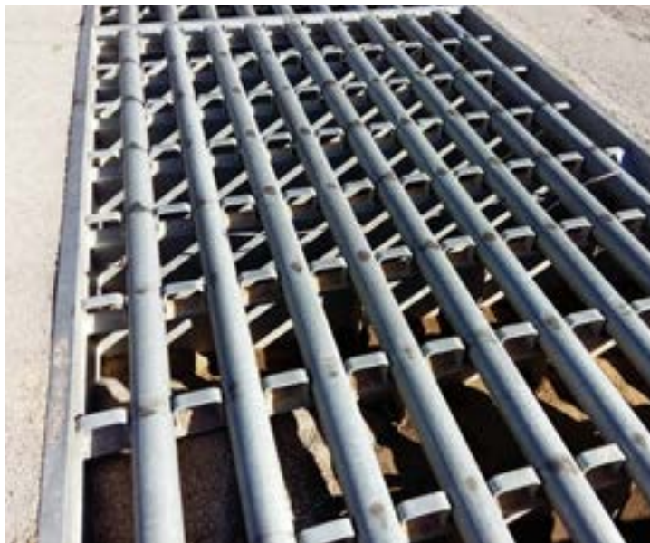
Figure 1.5. Cattle grid to prevent ungulates crossing intersections of fencing with paths.
