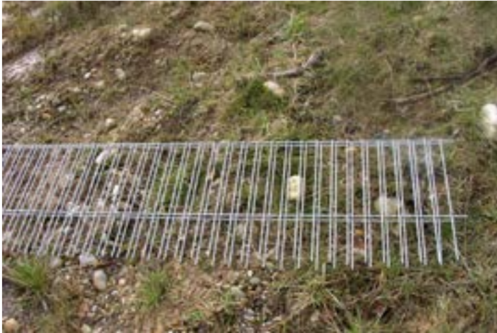
Figure 2.3. The horizontal wire at the base of the reinforcement mesh must be cut away to help stick the mesh into the ground.
