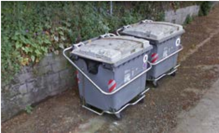
Figure 9.2. System of bars placed around containers to prevent them from being tipped.
