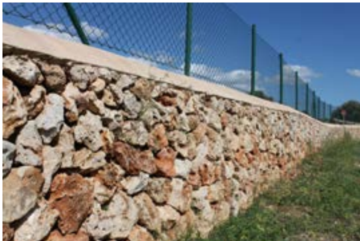
Figure 1.3. Stone wall suitable for blocking access of fauna, topped with a mesh fence to prevent access to people.
